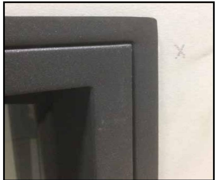
Figure 4.7 Front / Trim Ring Installed to Overlap Wall
