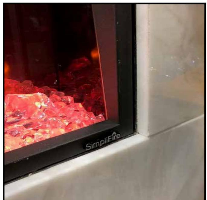
Figure 4.8 Front (without Trim Ring) Finished Inside Fit
