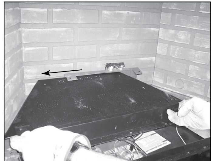
Figure 14.30 Side Burner Assembly to Left
