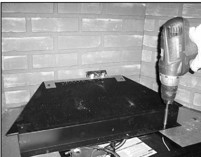
Figure 14.28 Remove Screws Attaching Front Burner Support
