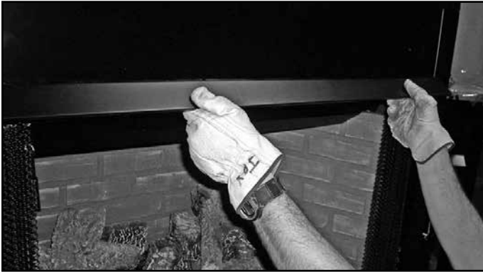
Figure 14.27 Installing the Hood
