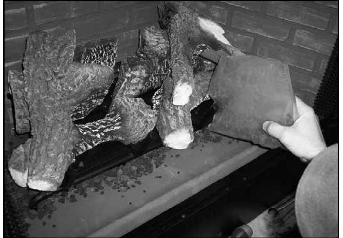
Figure 14.21 Placement of Lava Rock
