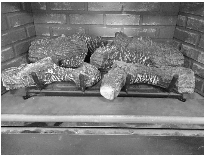
Figure 14.13 Left and Right Front Log Placement
