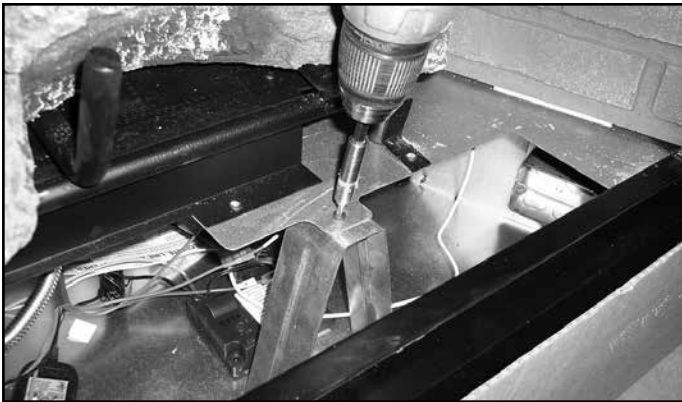
Figure 14.1 Remove Screw from Right Shipping Support
