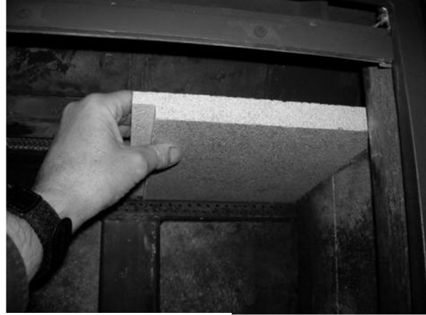
Figure 19b – Removing / Replacing the Baffle
