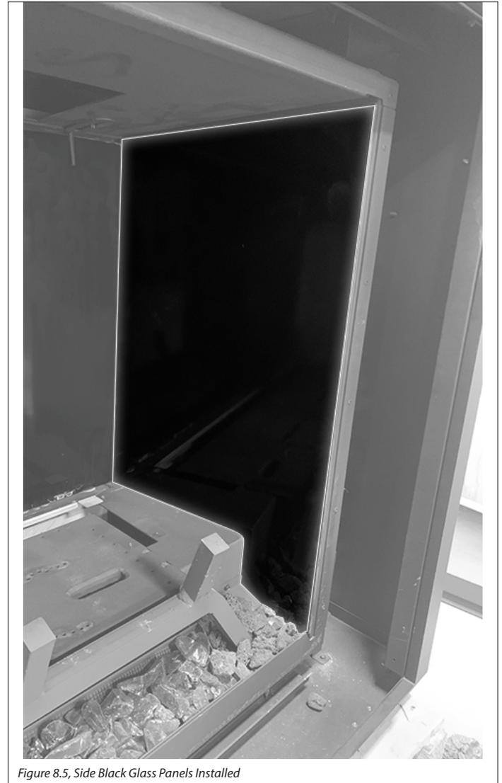
Figure 8.5, Side Black Glass Panels Installed
