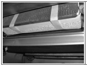
6. Since the combustor is only 2" deep, there is ample room to lift the new combustor into place. **REMEMBER TO HAVE THE TAB ACROSS THE BOTTOM EDGE OF THE COMBUSTOR AS IT IS INSTALLED**. Slowly push the combustor in at the top apply even pressure to the left and right corners. This will allow for a better view of the bottom edge for the final fitting. **DO NOT FORCE THE COMBUSTOR INTO THE DOME. TAKE YOUR TIME AND WORK IT INTO PLACE SLOWLY.**
